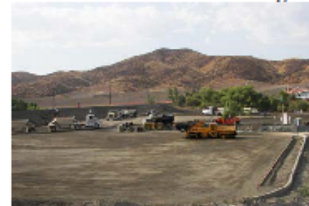
Today Machines working at Eastport
