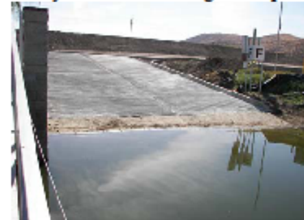
Eastport Launch Ramp poured last week
